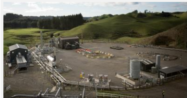
Underground gas storage
