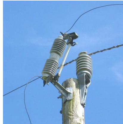
Fuses to more cheaply isolate smaller faults and lower voltages
