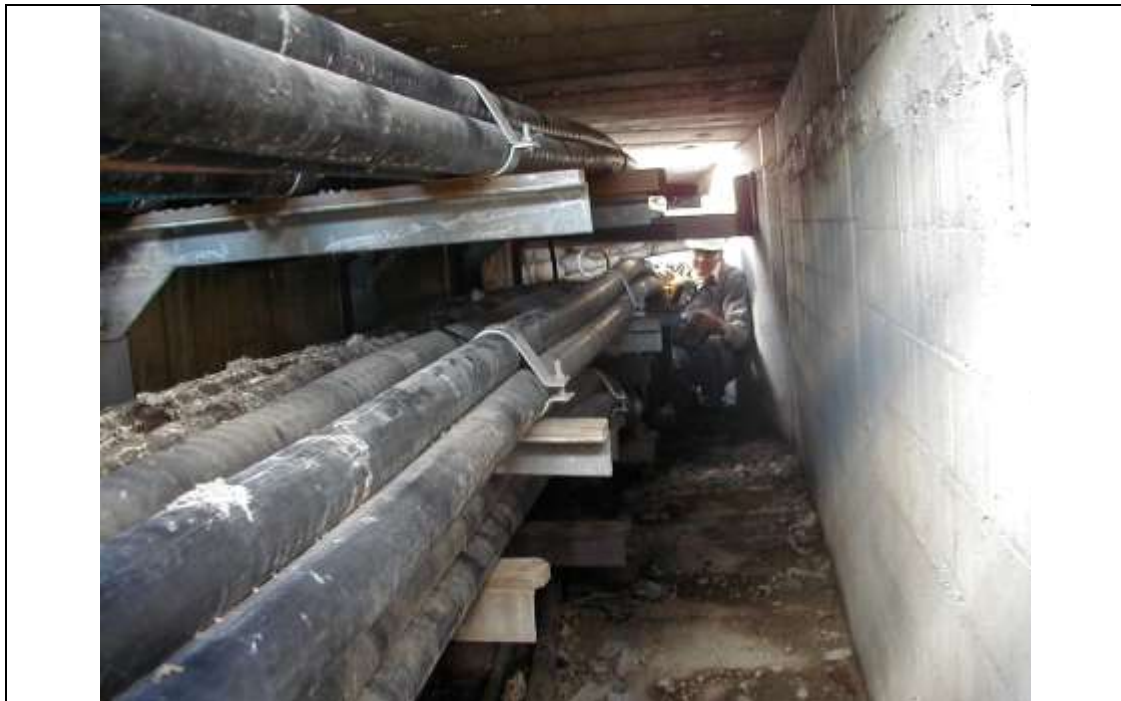
Figure 7 Photograph of the cable trench in 2001, near zero m, before the fire
