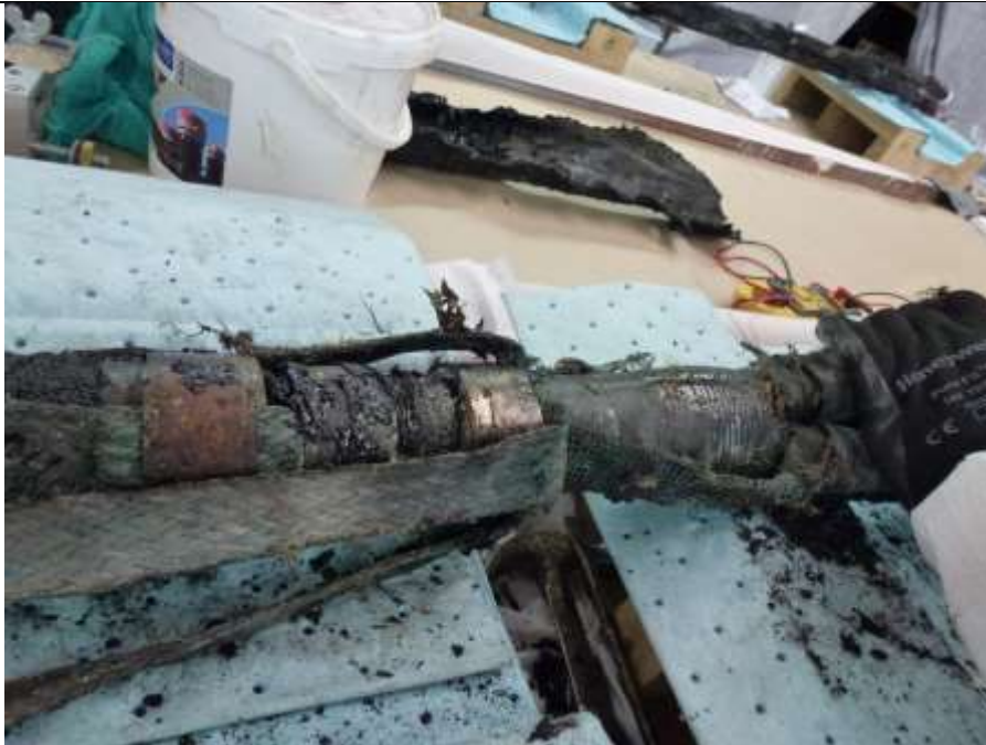
Figure 25 Unfailed joint. Outer heat shrink sleeve and copper mesh removed
