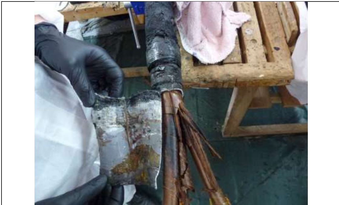
Figure 36 Black feature extends underneath and to the end of lead sheath cut
