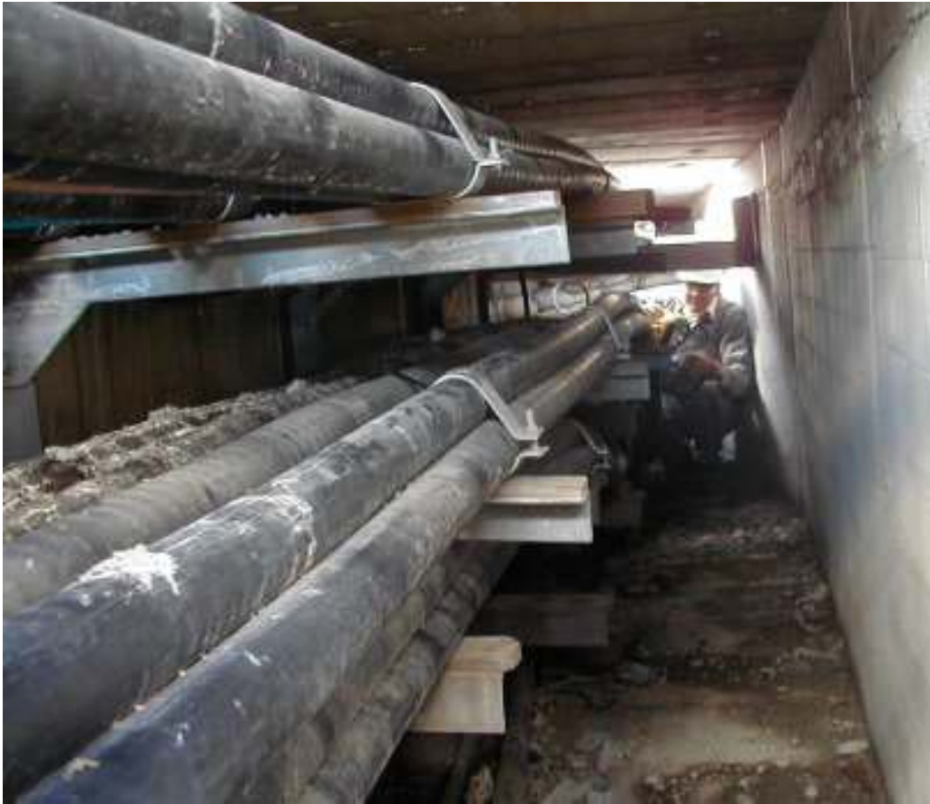
Figure 6 – Penrose cable trench in 2001
