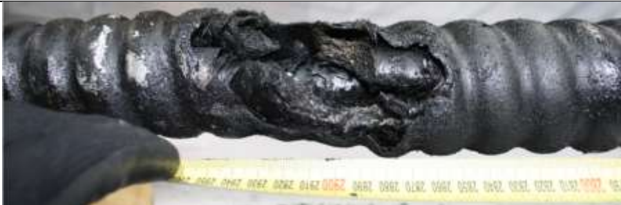
Figure 87 Arc crater: 33 kV OF, Carbine 1, 2DO, 68.9 m
