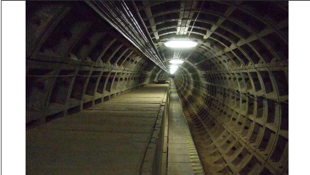
Figure 146 Wimbledon tunnel containing a cable trough
