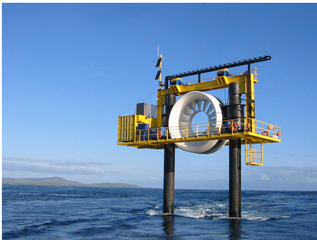
Figure 2.13: OpenHydro's Open-Centre Turbine at EMEC, May 2007 (© PPL)
